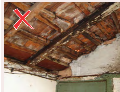
Damaged ceiling with water leaking
